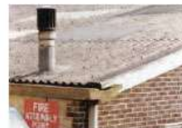
Asbestos cement roof
