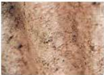
Sprayed coatings on ceiling walls, beams/columns
