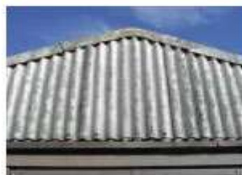
Asbestos cement wall panel
